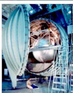
CRYOGENIC PROPELLANT TANK FACILITY
