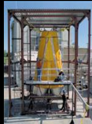
Cryogenic Propellant Tank Facility
