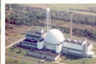
SPACE POWER FACILITY
